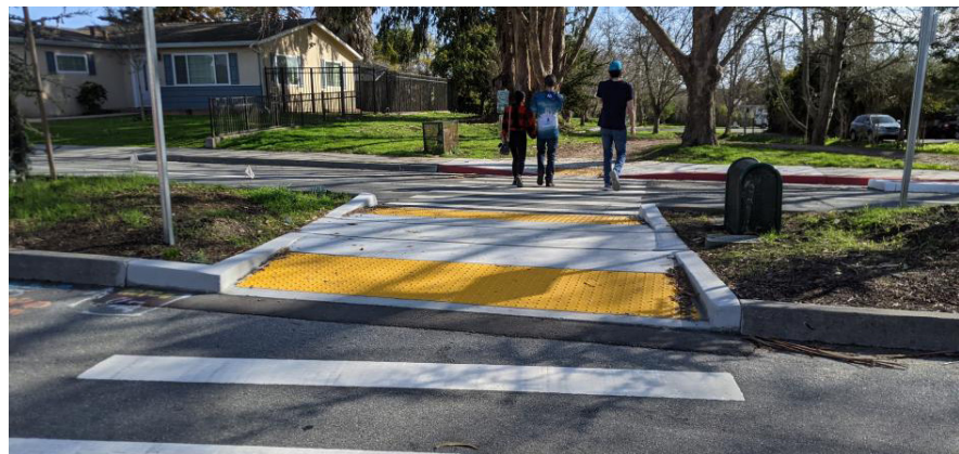
A pedestrian crossing with a refuge island enhances safety by increasing visibility to drivers and providing a safe midway point for pedestrians.
