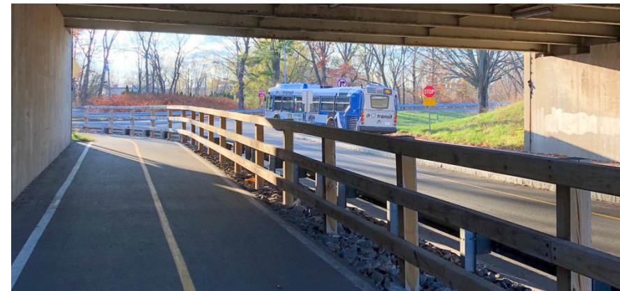
As the multiuse path travels underneath I-40, there appears to be room for a multiuse path under the existing bridge. However, the bridge could be rebuilt (in the future NCDOT STIP process) to accommodate a wider, more comfortable facility.
