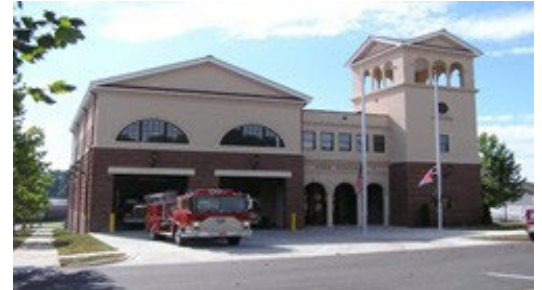
Fire Station #3 Building
